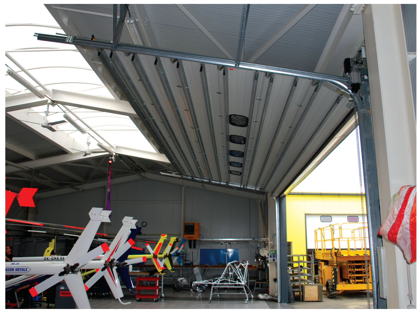
FSL Standart Lift under 15° angle
